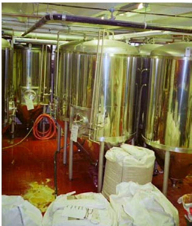
Pipeless CCT installation at the old location at Kungsholmen
