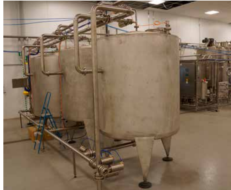
CIP unit Wellnox under installation
